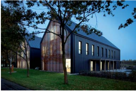
Figure 5 Photograph of the building, as built, taken from west facing towards east.
